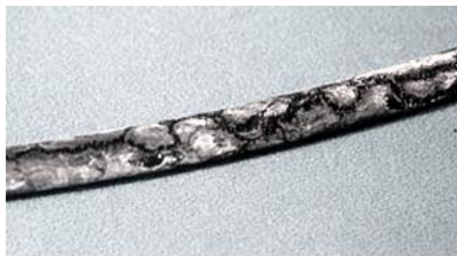
Fig.1: Surface tracking of conductor insulation.
